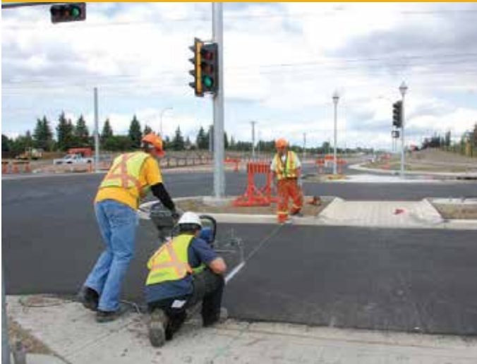
STEP 1: Pre-marking the lines
