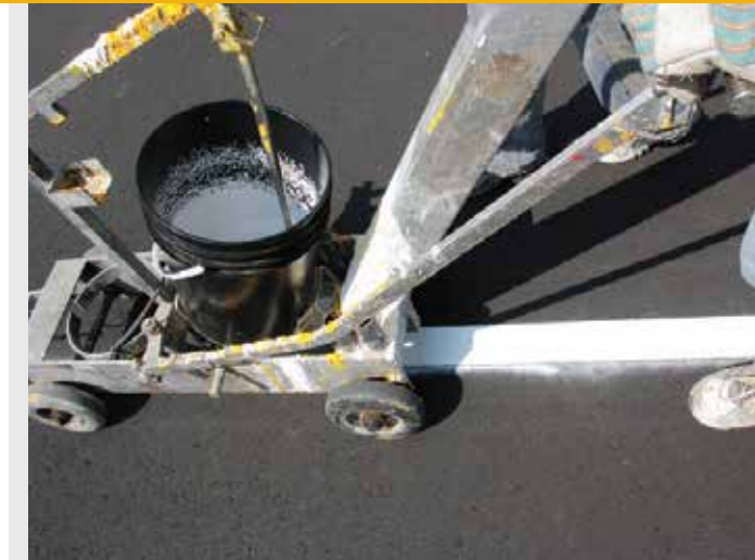
STEP 4: Longitudinal line application
