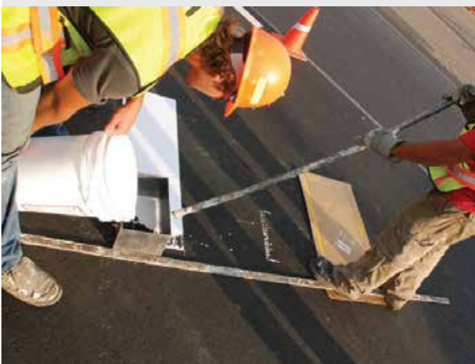
STEP 3: Stop-bar application
