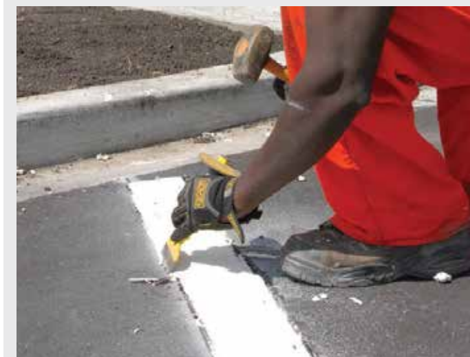
Trimming a line for quality control
