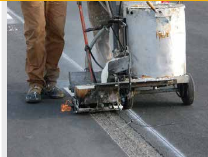
Longitudinal line application
