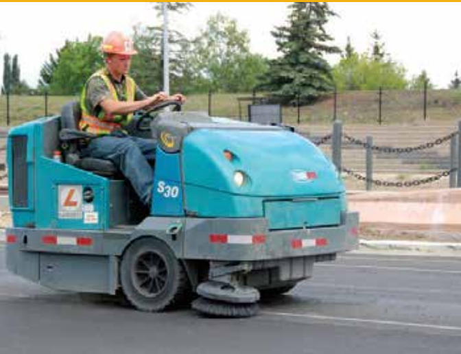
Cleaning the road surface
