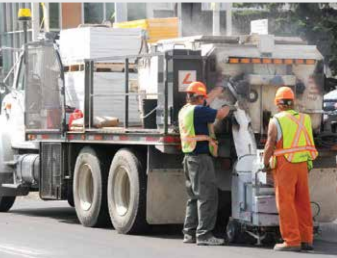
Transferring plastic to the applicator
